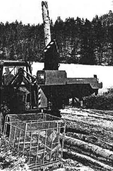
● The unparalleled firewood processor, hands-free operated from tractor seat, - feeds, cuts and splits logs with no direct physical intervention by the operator (patent pending). The machine took a silver medal at Agritechnica '99 in Hannover, Germany.
